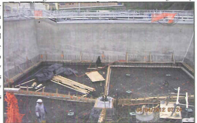
Construction of the Clarifier Underway
